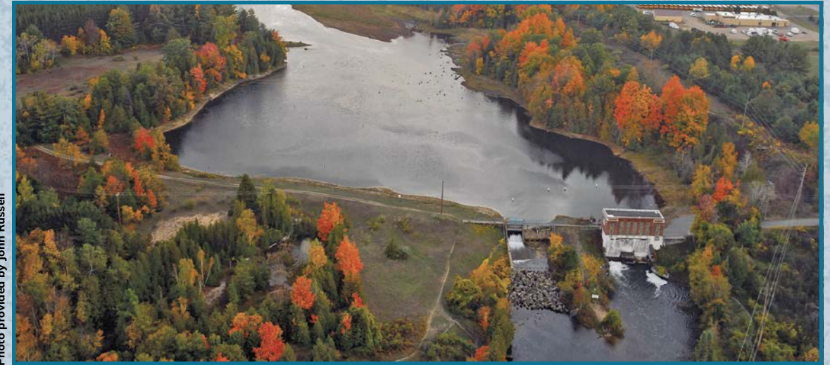
Underneath Sabin's impoundment were years of accumulated sand and sediment. All sediment was kept on-site and smoothed into adjacent upland areas outside of the river channel and its floodplain. (October 2012)
