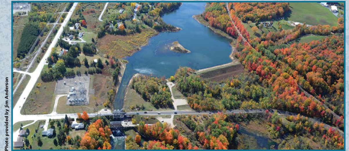
The Boardman Dam impoundment. Note the powerhouse and dam, called the core wall, are separate structures. (October 2016)
